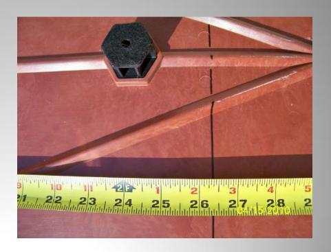
26 3/8" on a 2x5 tile will cut thru the center of the plus and leave all anchors in place. No anchor moving necessary.
